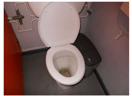
Photo 21 - Typical WC pan.
