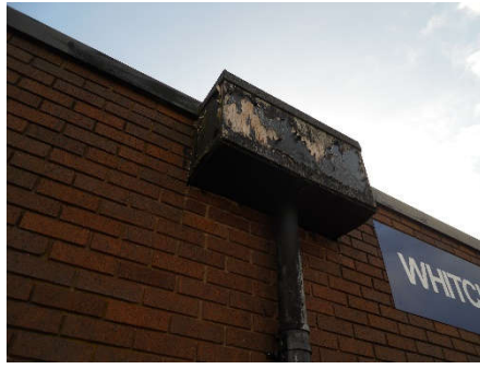
Photo 23 - Rainwater down pipe and hopper head detail.
